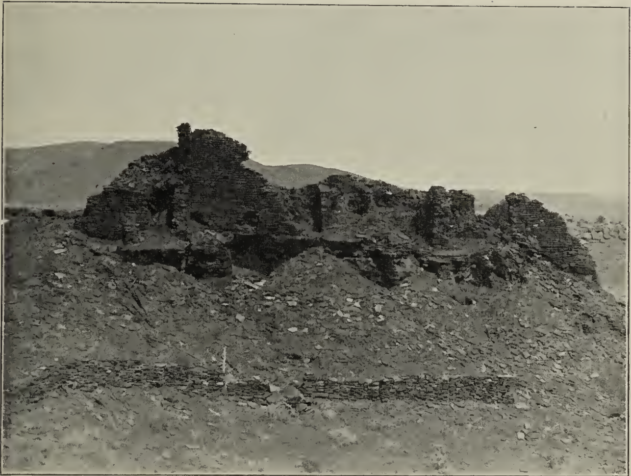
VIII. VIEW OF SECTION A OF WUKOKI; SHOWING MODERN STONE WALL IN THE FOREGROUND, AND DEBRIS AT BOTTOM OF THE MESA
